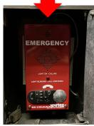
For the Cohen Garage, there are call buttons in both elevator cars that will ring directly to Schindler Elevator in case of entrapment.
